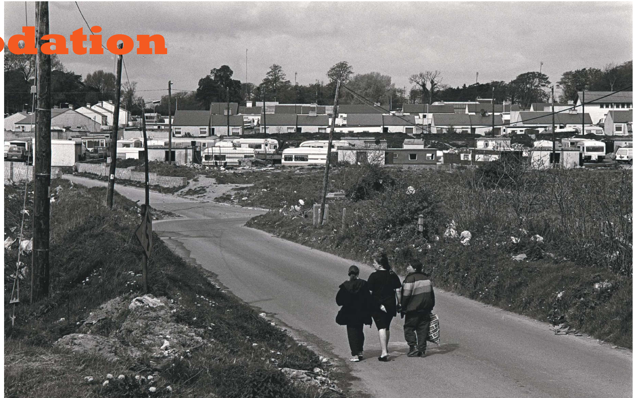
April 1994, Cara Park Group Housing and Halting site, Coolock, Dublin.
